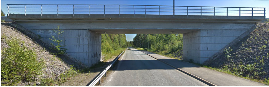
Figure 10: Hörnefors railway bridge.
